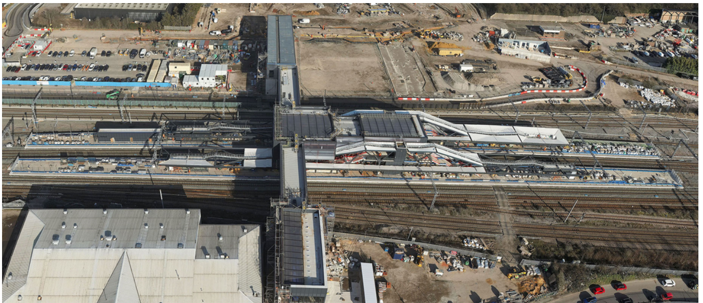
Brent Cross West Station February 2023)
