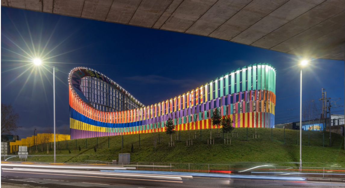
Brent Cross Town primary substation
